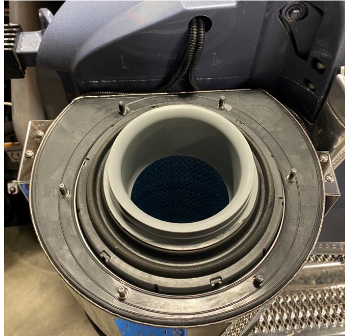
Figure 10: Wiring Harness Tucked Between Air Cleaner and Plastic Panel (Driver Side Shown)
